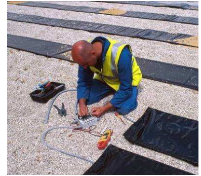
Connecting pads to a terminal box
